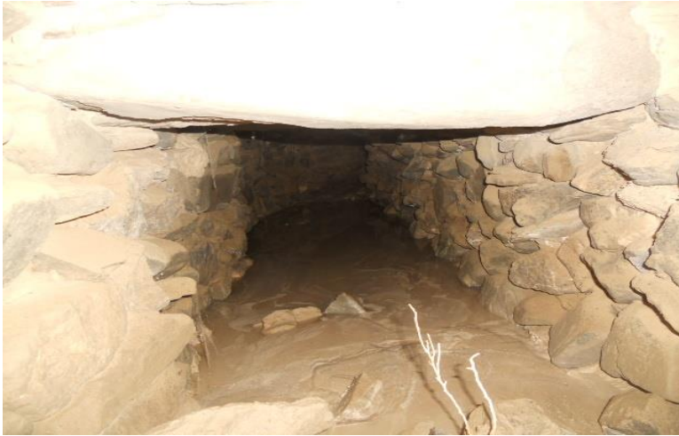
Tunnel in Khazanagi Bhutt near Reko
